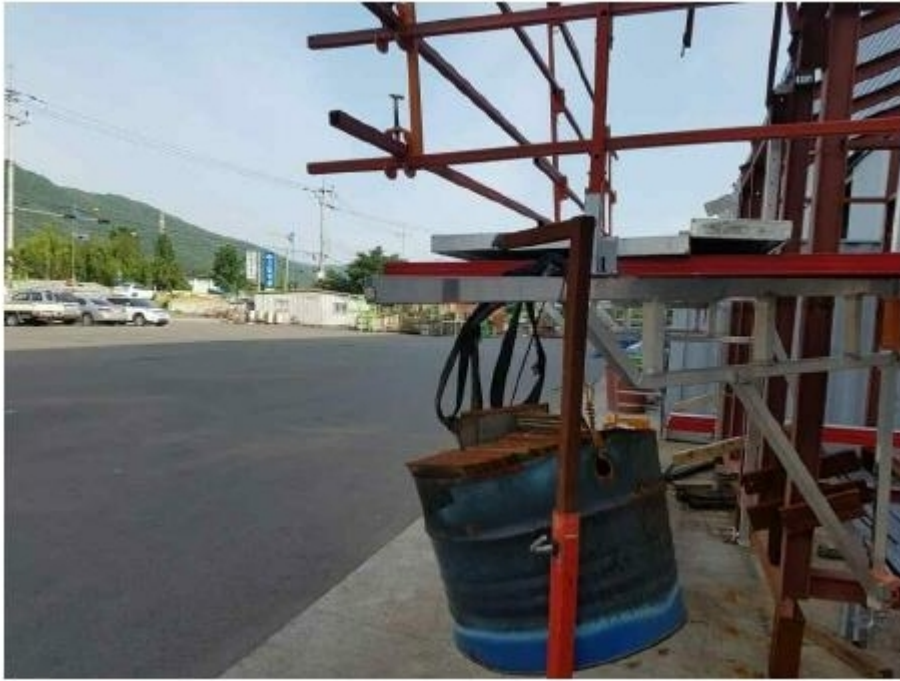
Figure 8- Static Load 339 KGF at 2.2 meter Corner Arm
